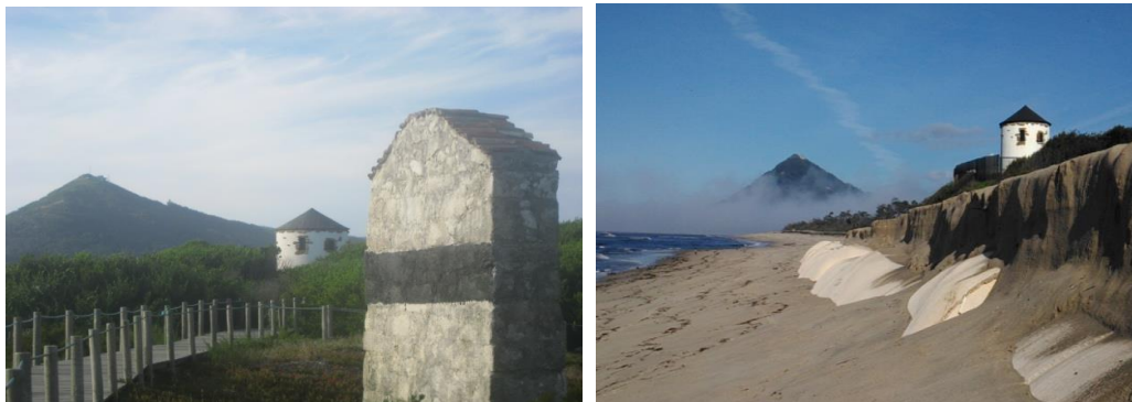
Figure 14 - Aspect of Moledo do Minho beach area in August 2009 (left), before the 2014 'Hercules' storm, with a stone wall and wooden walkway (overthrown meanwhile) and the Mill surrounded by vegetation. The same place in December 2019 (right) after a storm which was partially exposed a geotextile tube previously installed there.
